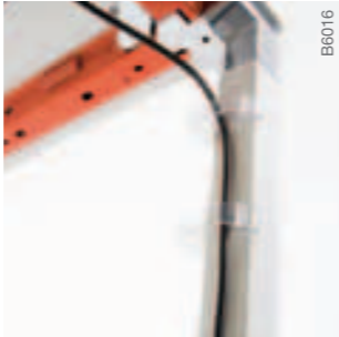
Cable clips, translucent plastic, attached to leg.
